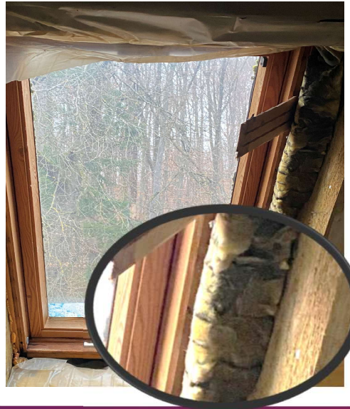
Undichte Fensteranschlüsse
